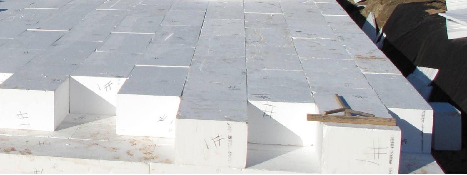
GeoFoam being laid in a brick pattern. Installed fit for fit.
